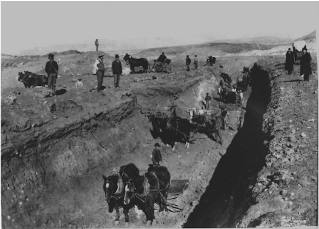
Construction on Saint George and Washington Irrigation Company Canal
