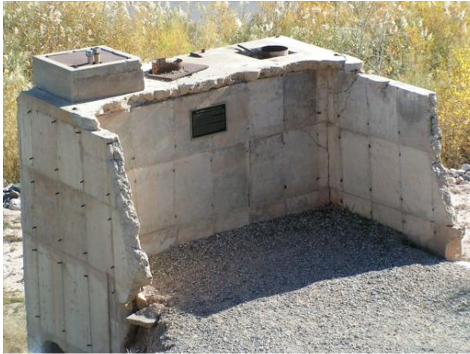
Virgin River Pump Station 2010
