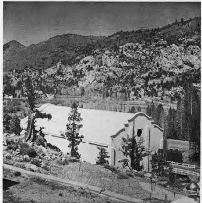
Rush Creek Plant Mono Basin, California
