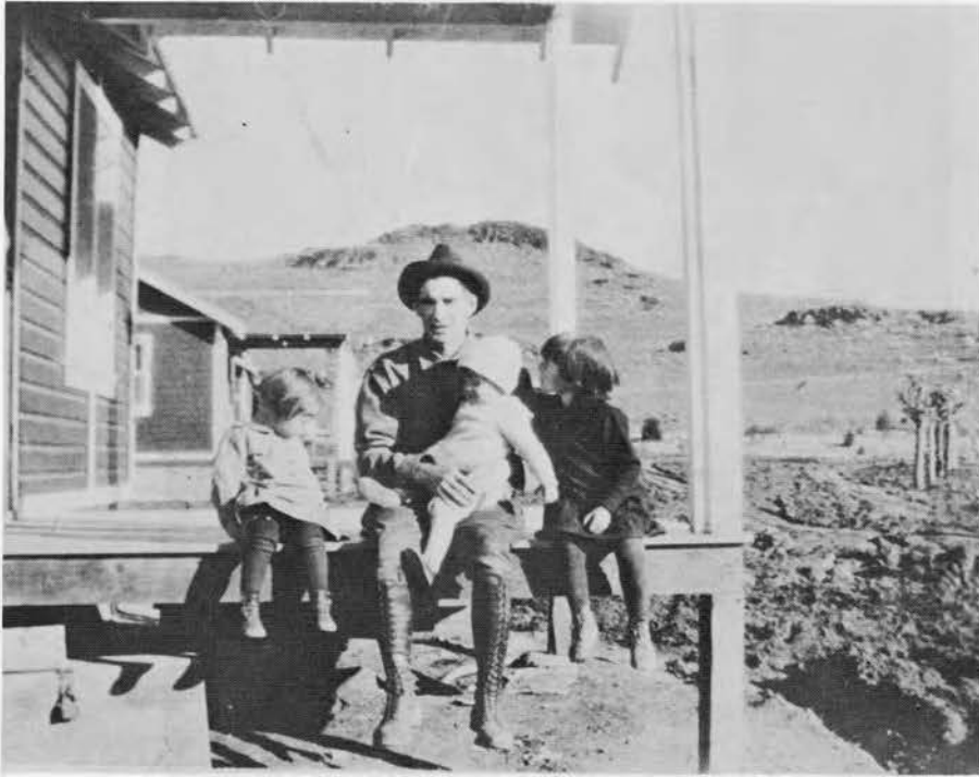
#3 Hydro Plant, just completed Alice, Vaughn holding Maurine, LaVerne
