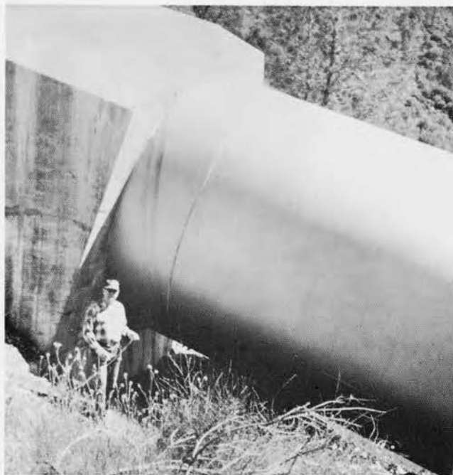
Emerald Seitz by pipe powerhouse #4 Big Creek, California
