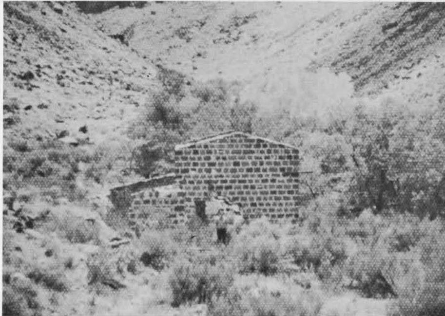
Old #1 Power Plant on Santa Clara River between Gunlock and Veyo
