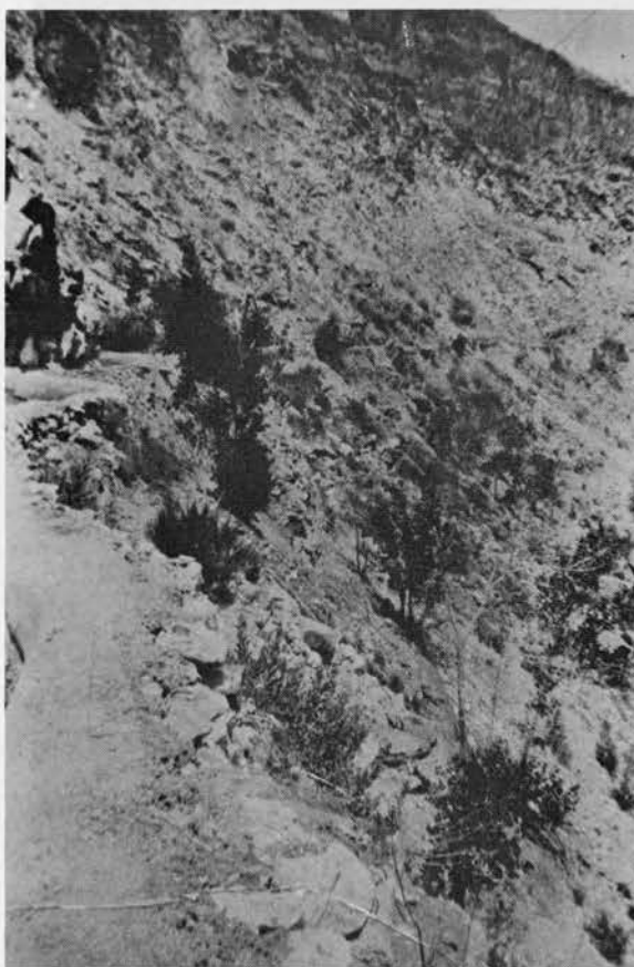
Canal to Hydro Plant #4 LaVerkin, Utah
