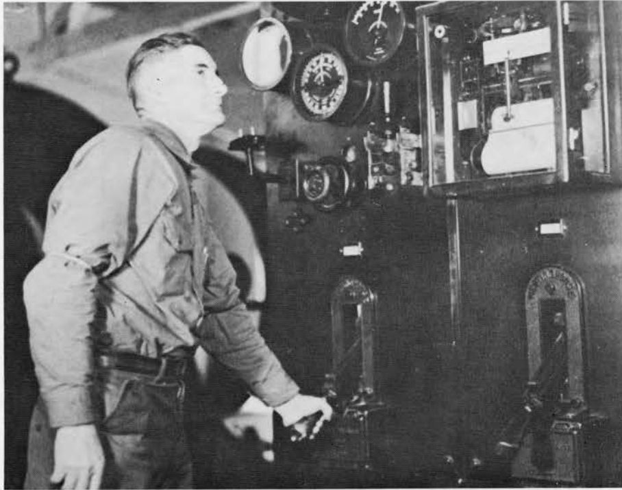
Vaughn at Controls #3 Plant
